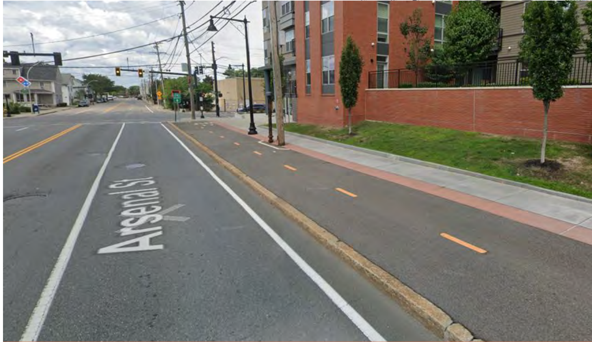
Arsenal Street Cycle Track is proposed to extend to the Taylor Street path
